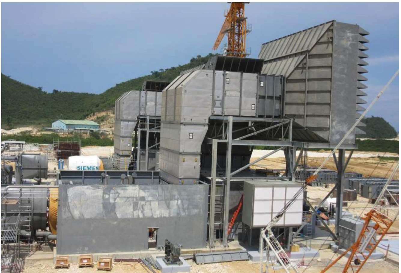
Construction of Power Station
