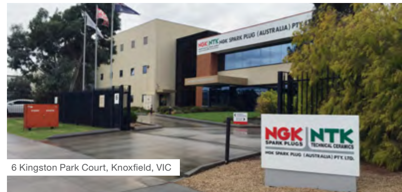
1500 Ferntree Gully Road & 8 Henderson Road, Knoxfield, VIC
