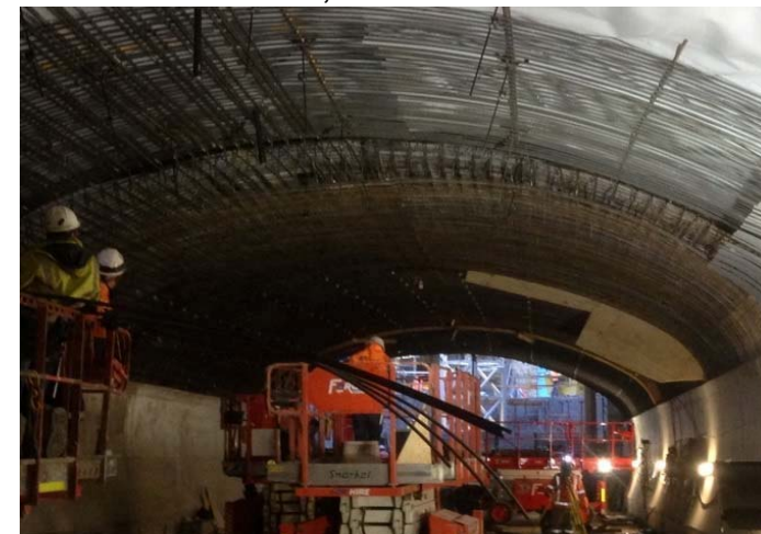
Wynyard Tunnel, NSW
