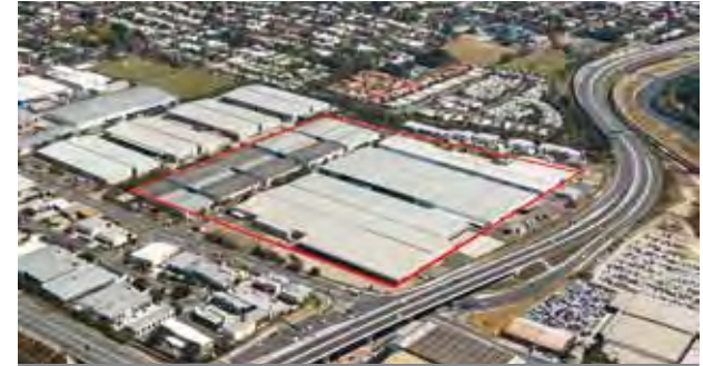
Hendra Distribution Centre
