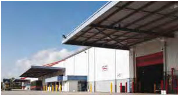
Forrester Distribution Centre
