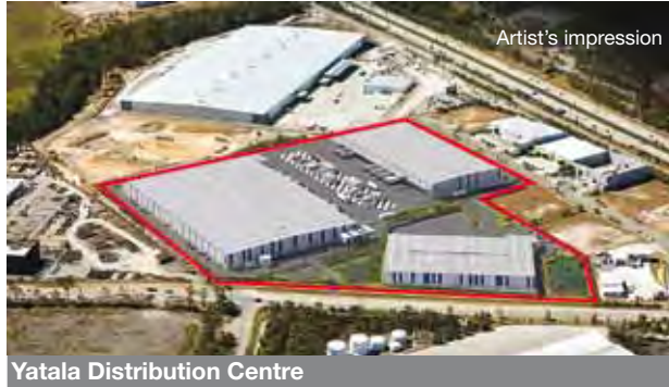
Yatala Distribution Centre
