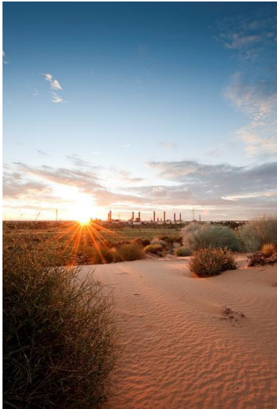
Moomba Plant, Cooper Basin
