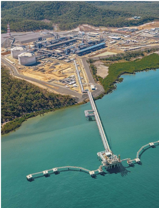
GLNG plant, Curtis Island, July 2015
