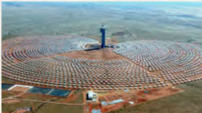
Solar thermal tower project, South Africa.
