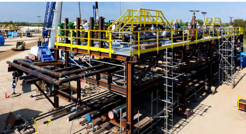
WorleyParsonsCord, Blackfalds Module Yard, Canada
