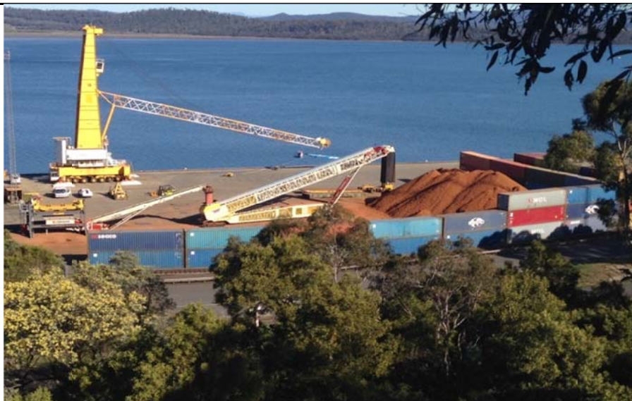
Figure 11 Overview of bauxite stockpile at Berth 5, Bell Bay Port
