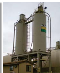
Fly ash terminal - Denver
