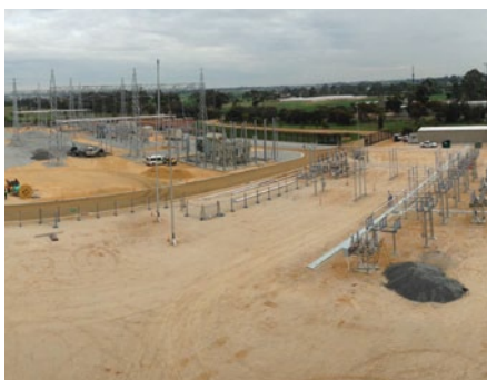
Image on top: CaMS City West Substation. Middle: CaMS NBN Warehouse. Bottom: Munno Para Substation being built.
