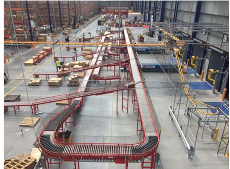
New Australian National Distribution Centre
