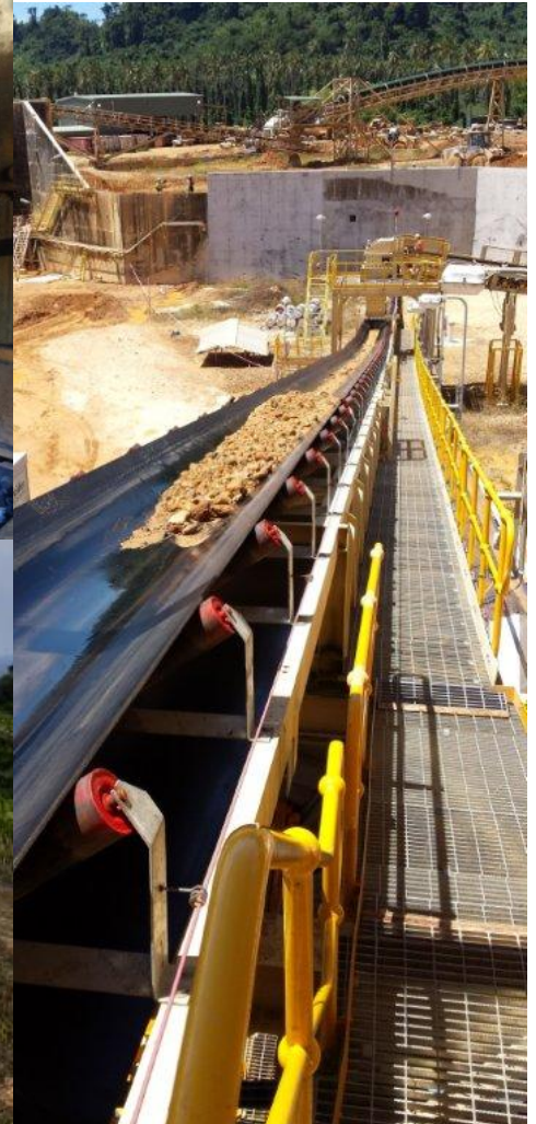
SAG Mill Feed Conveyor
