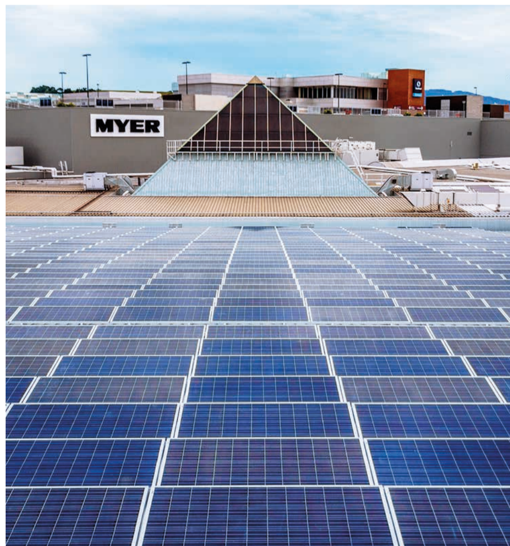
Stockland Shellharbour rooftop solar, NSW.
