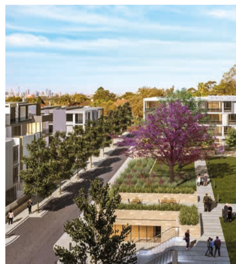
Cardinal Freeman Retirement Living Village, under construction in Ashfield NSW.
