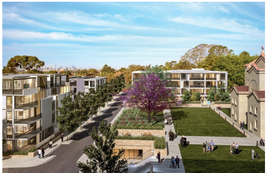
Cardinal Freeman Retirement Living Village, under construction in Ashfield NSW.
