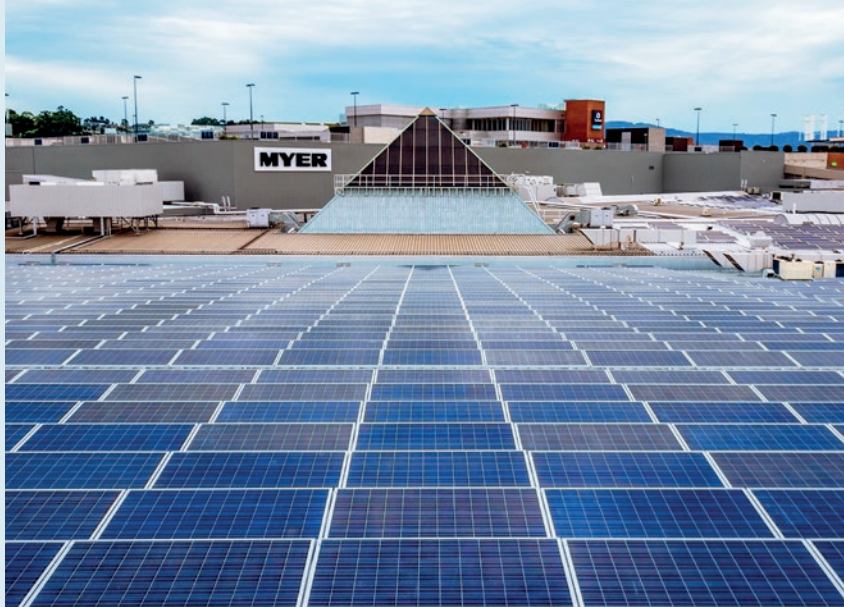
Stockland Shellharbour rooftop solar, NSW.
