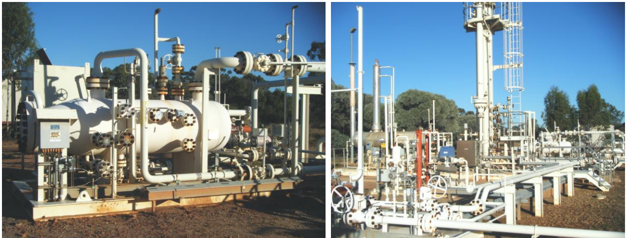
Gilmore Gas Plant, Australia
