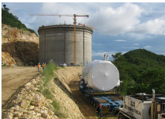
Unloading of Gas Turbine
