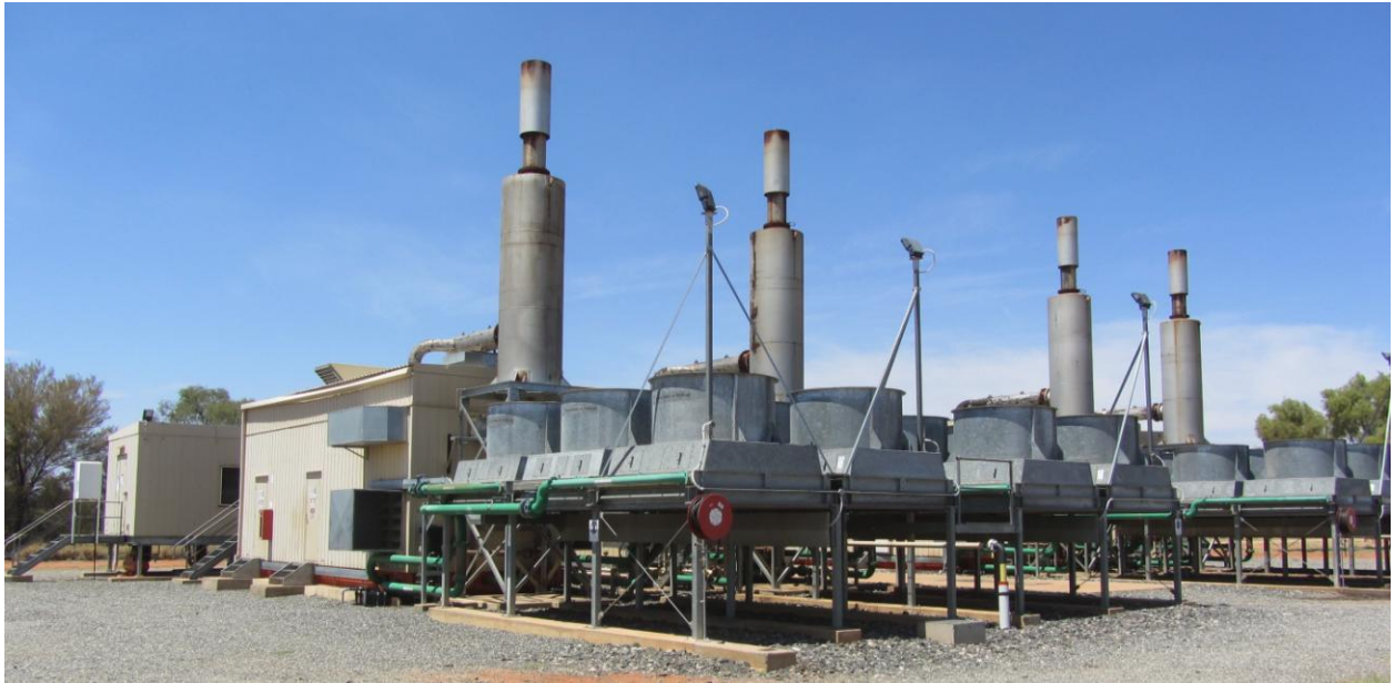
Alice Springs Power Plant, Australia
