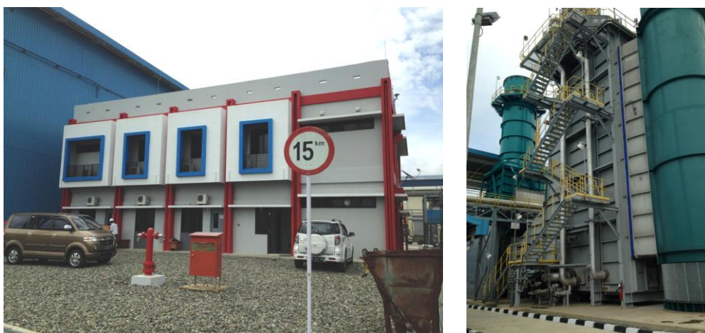
Sengkang Power Station in South Sulawesi, Indonesia
