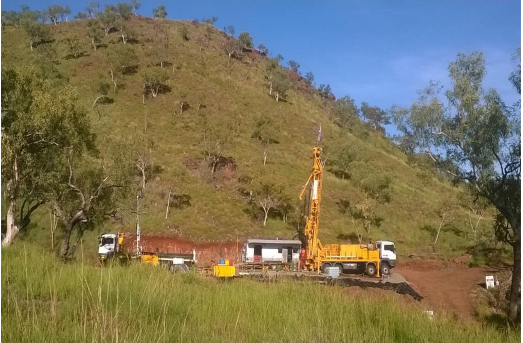
Surface drilling at Savannah North
