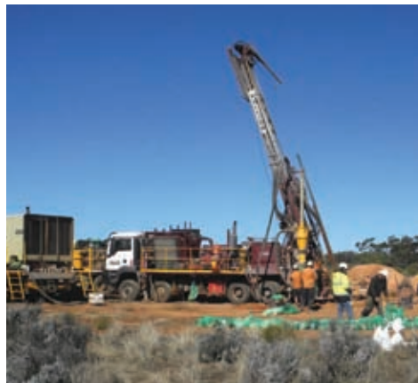
Drilling near Paris Project.
