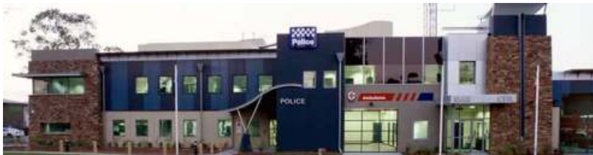
An example of Strata PNA's work - Diamond Creek Police Station
