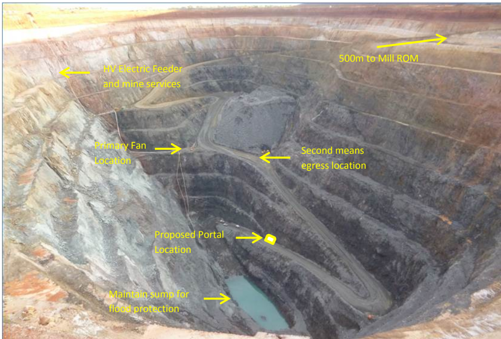
Figure 11 – Whirling Dervish Open Pit (looking north) showing proposed Portal location and general infrastructure
