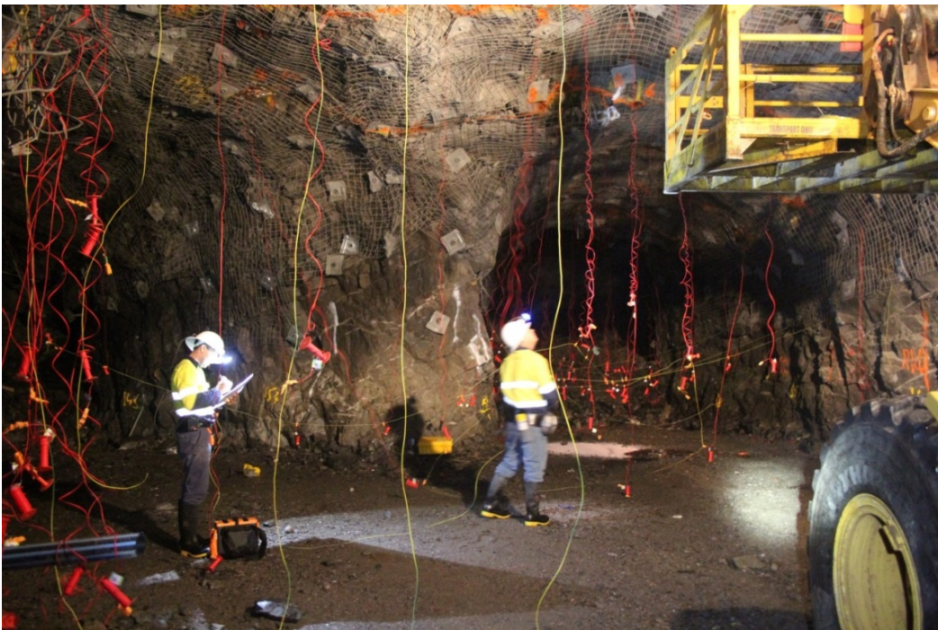
Figure 10 - Stope Charging Karari Underground 2190 Hangingwall lode
