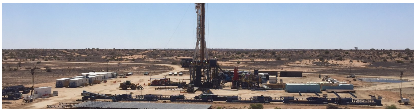
Drilling commenced at the Efficient-1 well site in October as part of the unconventional gas exploration program with Origin Energy
