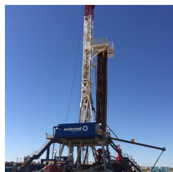
Easternwell Rig 106 mobilised to the Efficient-1 gas exploration well site (Origin Energy joint venture)
