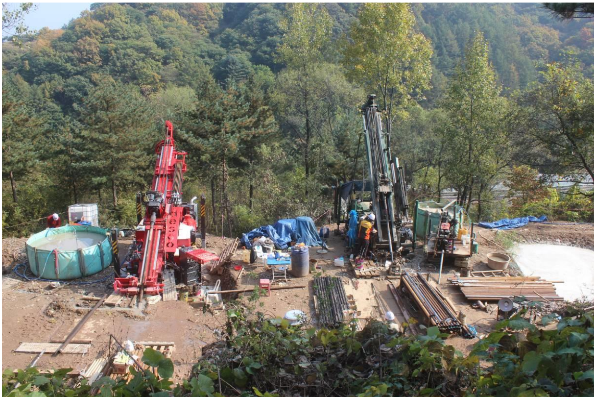
Figure 7: Rigs drilling holes DW009_2014 (RHS) and DW007_2014 (LHS) on section 5.
