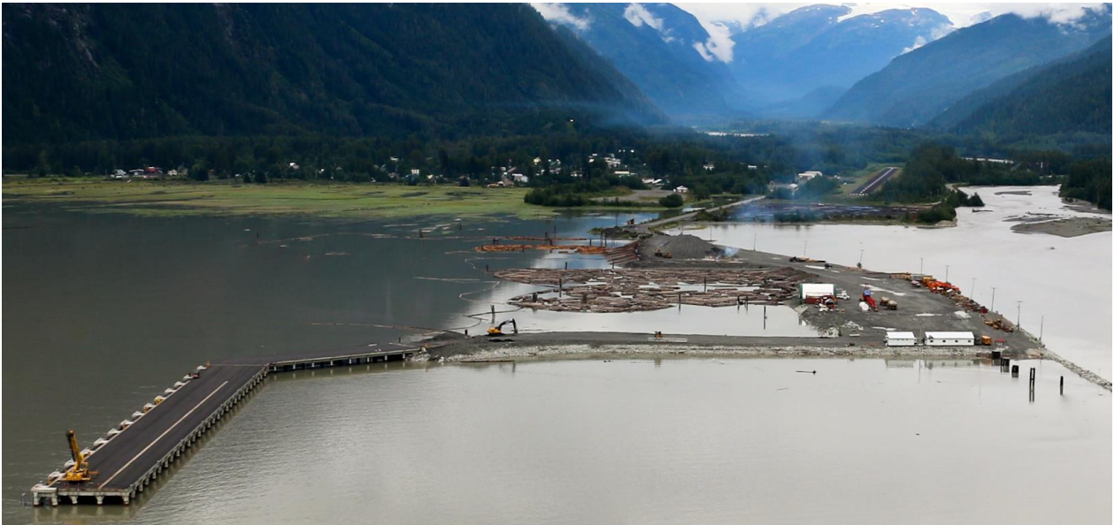
Plate 3. Stewart World Port – Berth Completed September, 2015
