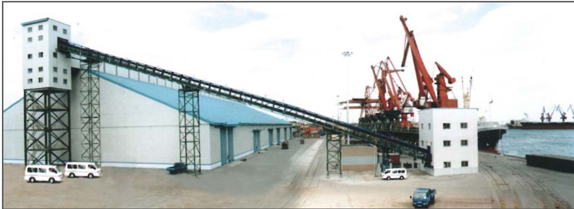
Bulk Handling Port Facility, China – Design/Build by FHC
