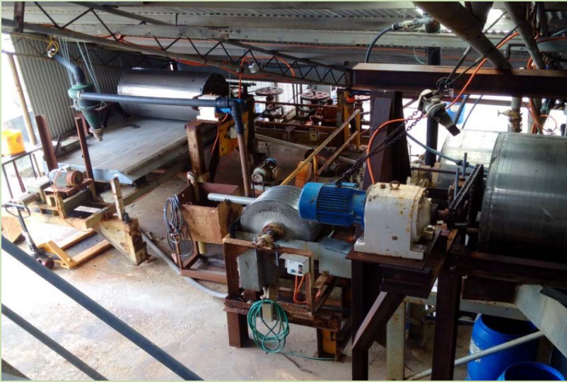
Re-start Processing plant (grinding, gravity, flotation)
