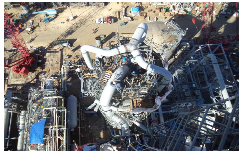
Piping being connected on the top of Stripper Column
