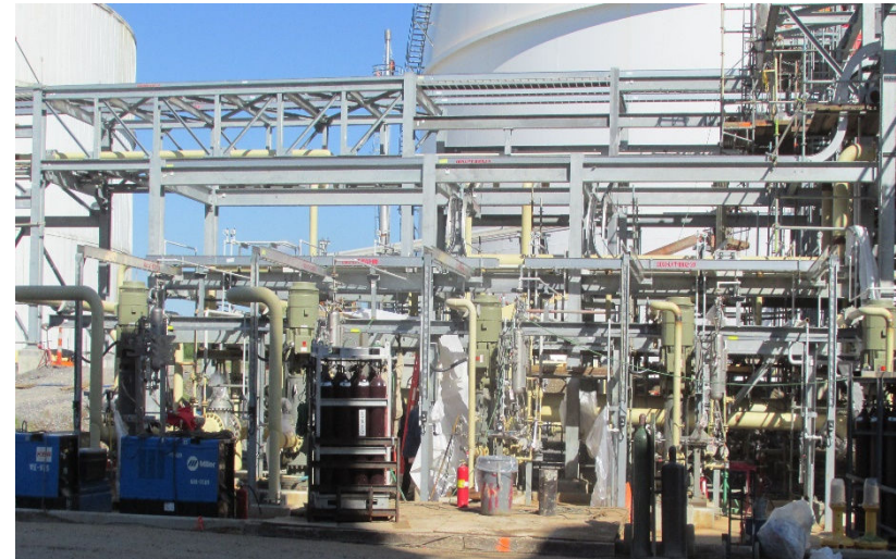
Ammonia loading pumps system being completed
