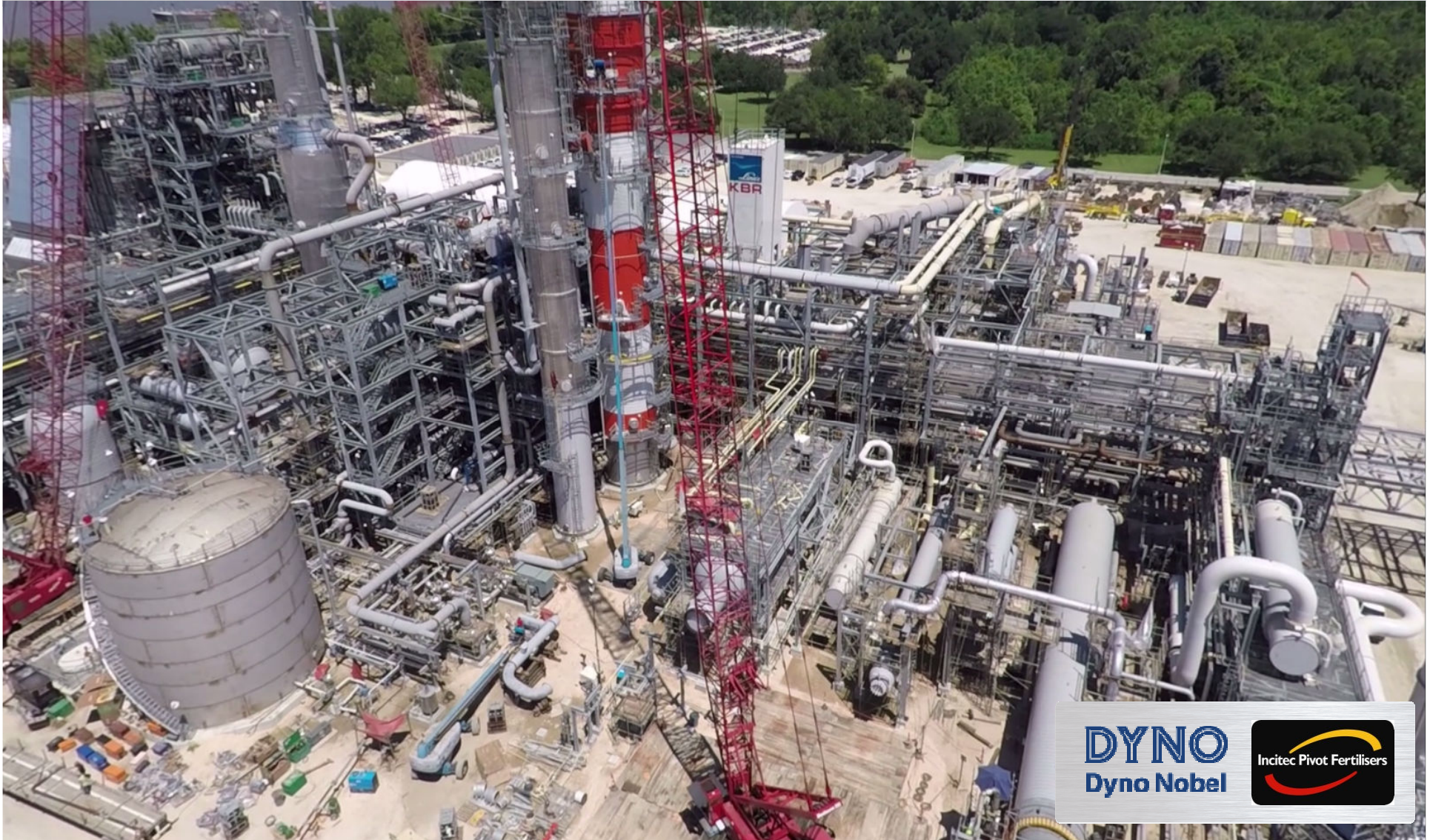
WALA ammonia plant under construction
