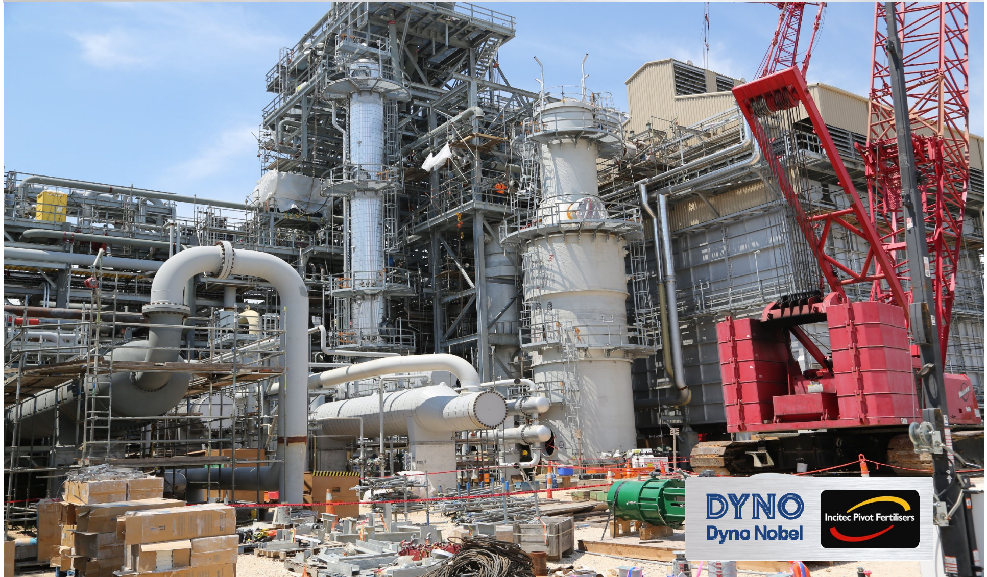
WALA ammonia plant under construction
