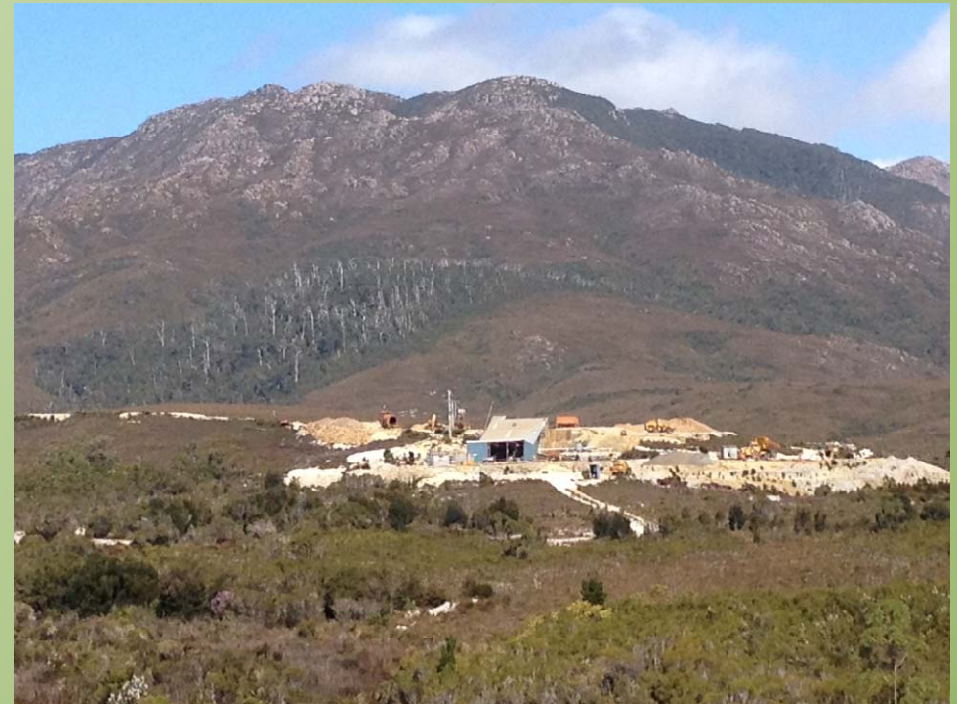
Granville Processing Plant in foreground Mt Heemskirk in background
