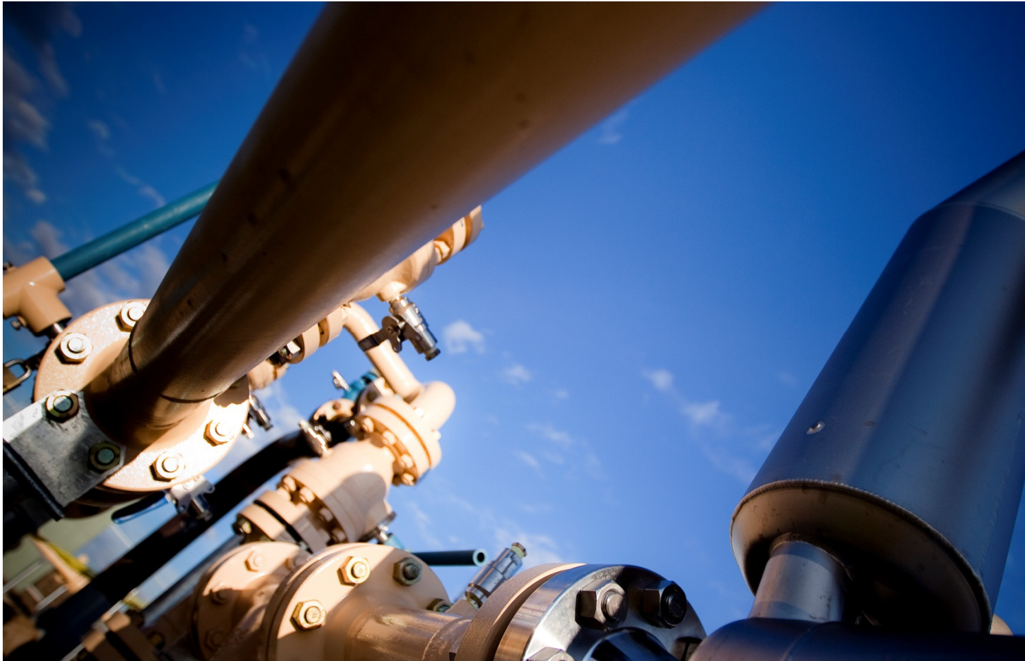
Pressure reduction station
