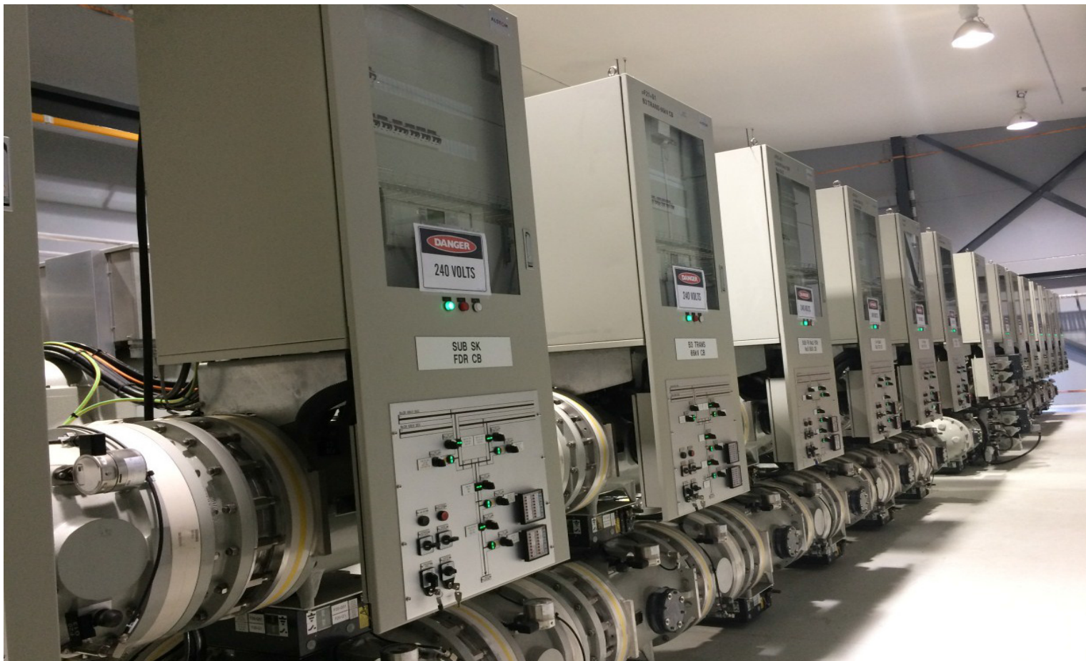
New indoor 66kV Gas Insulated Switchgear at Richmond Terminal Station
