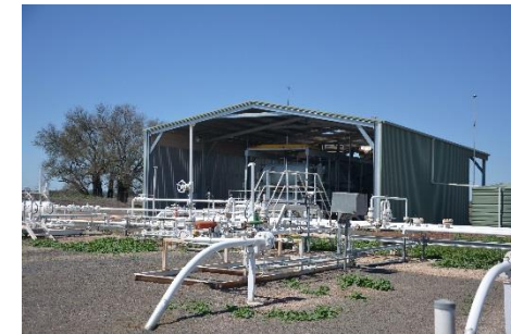
Myall Creek compression facility
