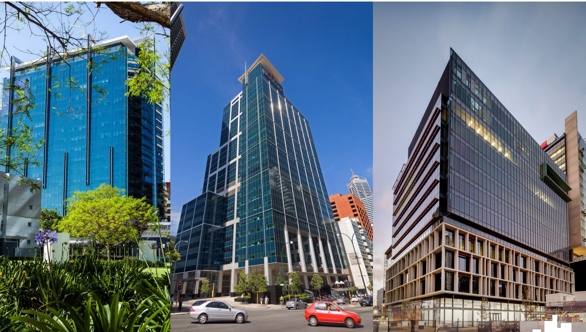
L-R: 58 Mounts Bay Road, 240 St Georges Terrace and Kings Square development, Perth, WA.
