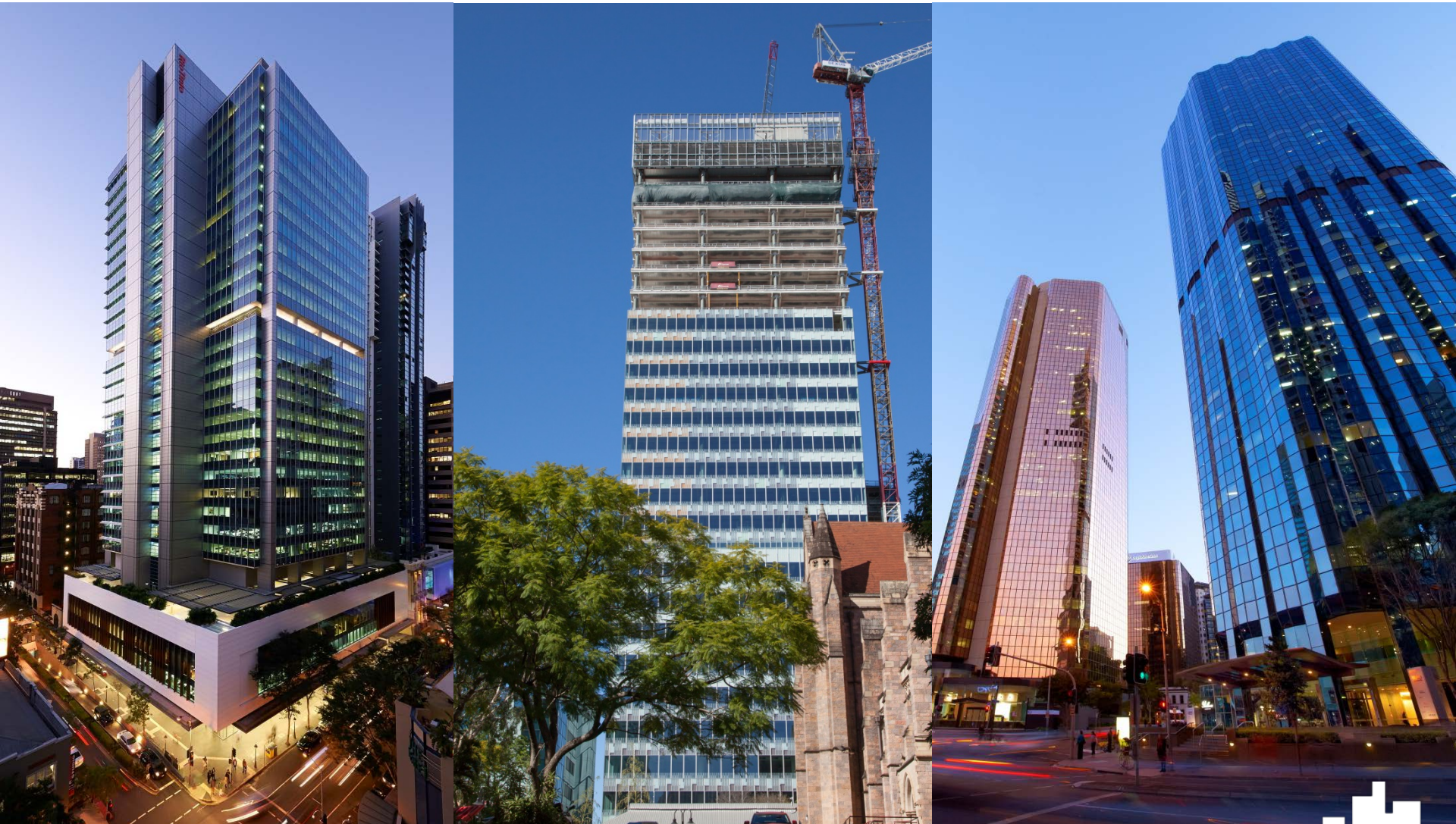
L-R: 123 Albert Street, 480 Queen Street development, 10 Eagle Street and 12 Creek Street, Brisbane, QLD.
