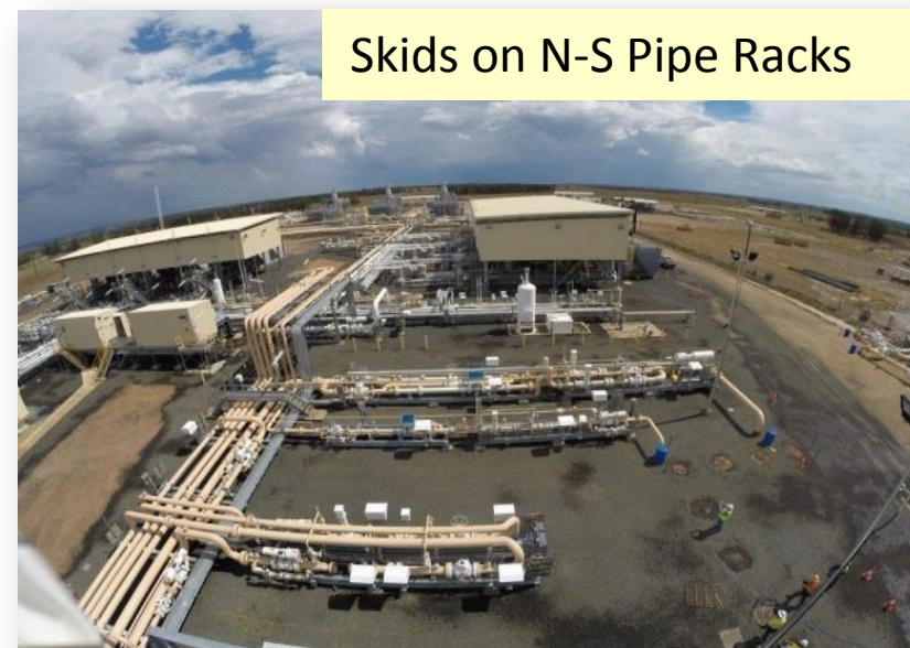
Lower – BWP Flow Reversal Skid
