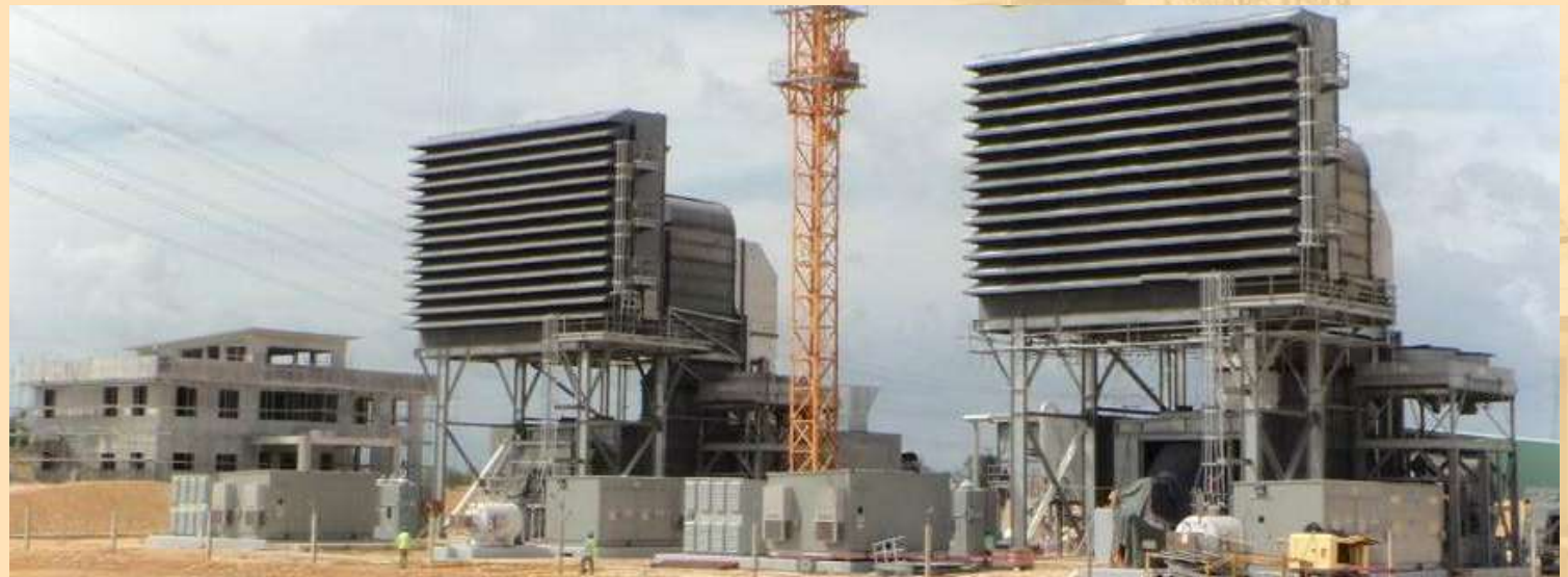
Power Plant in November 2015
