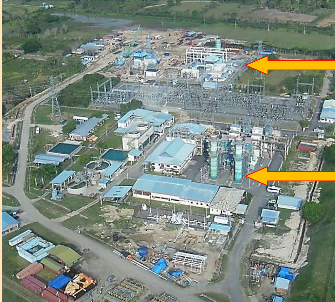
Aerial view of Sengkang Power Plant
