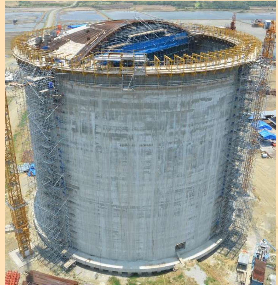
LNG Tank in October 2014
