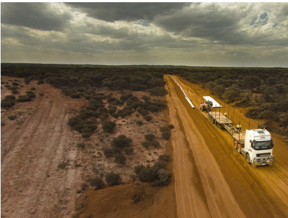
Figure 10 – Establishment of pipelines
