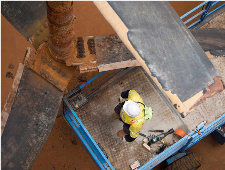
Figure 7 – Leach tank agitators
