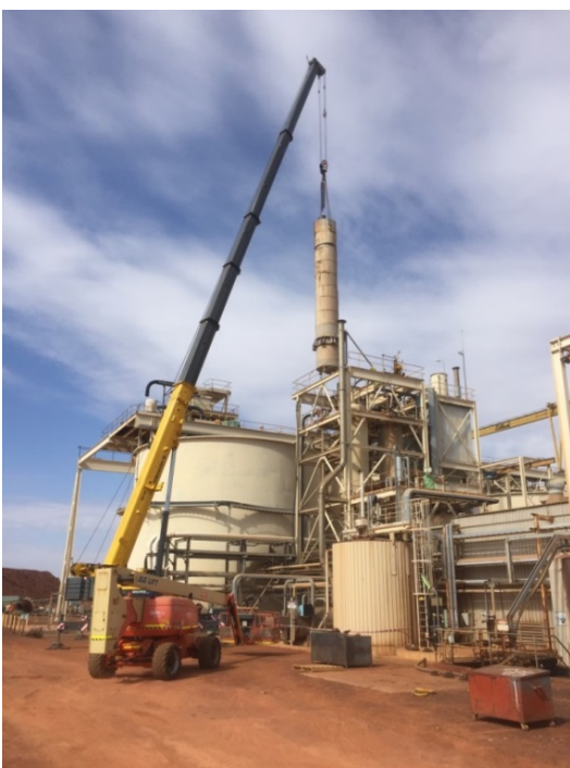
Figure 8 – Placement of elution column
