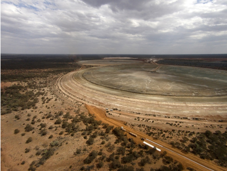
Figure 9 – Thunderbox tailings storage facility
