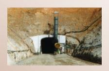
**Decline ramp provides Capex** efficient access, ventilation and haulage route
