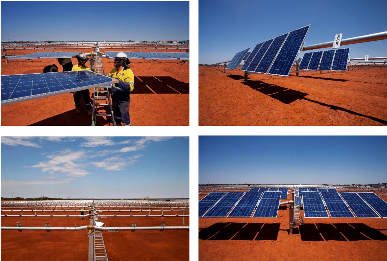
Figure 3 – Installation of photovoltaic panels at the DeGrussa Solar Power Station
