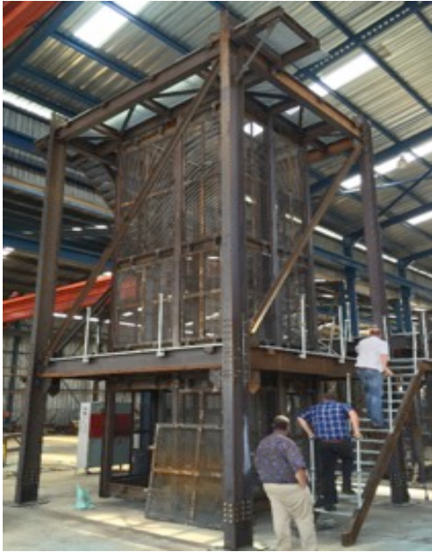
Photo 4. Headframe trial assembly - mid-section
