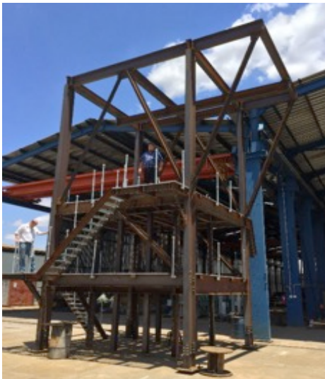
Photo 5. Headframe trial assembly - top section
