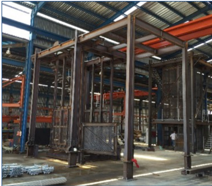
Photo 3. Headframe trial assembly - base section
