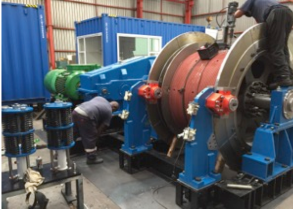
Photo 1. Main Winder undergoing inspection after trial assembly
