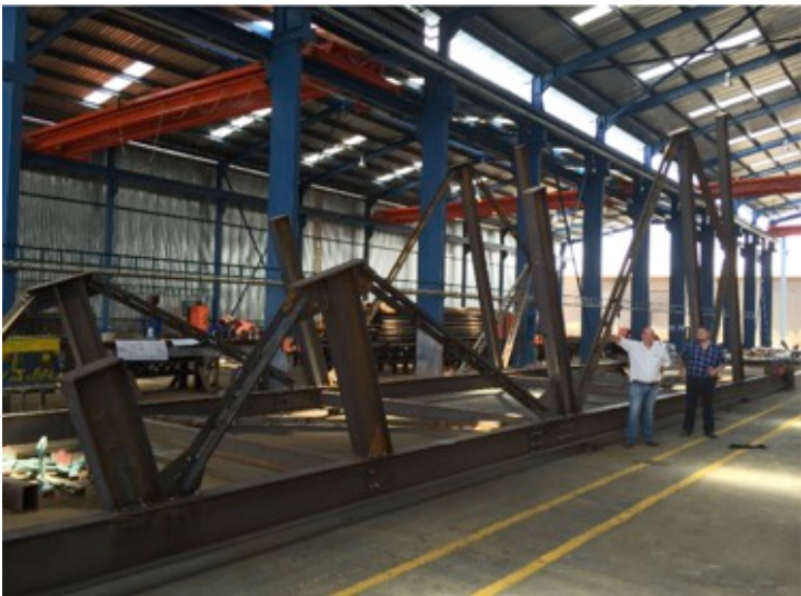
Photo 6. Headframe trial assembly - raker legs
