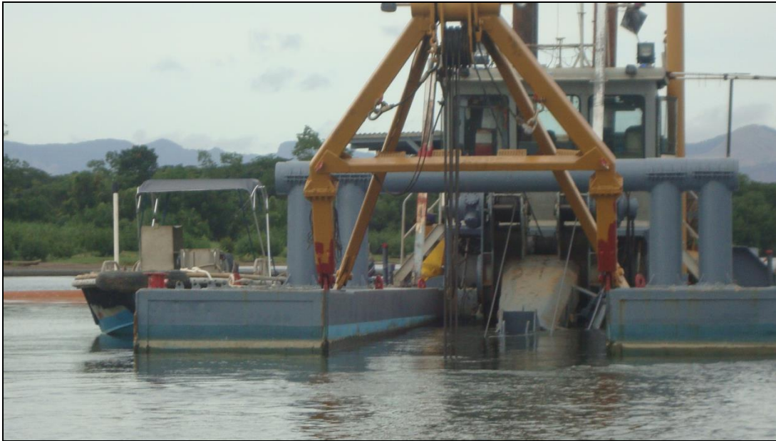
Ba River Dredging Operations
