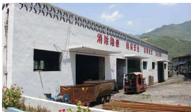
Fig. 9 Repair Workshop and Storage of Caotang Mine
