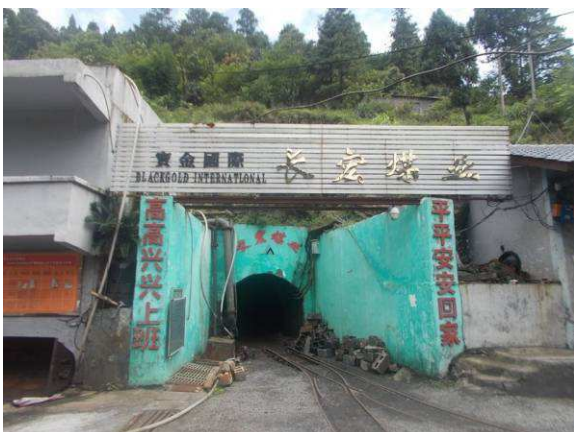
Fig. 21 Primary Transport Adit of Changhong Mine
