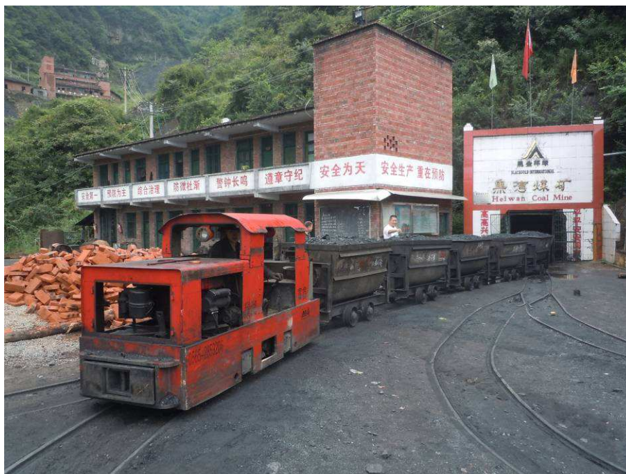
Fig. 12 Locomotive for tub haulage of Heiwan Mine
