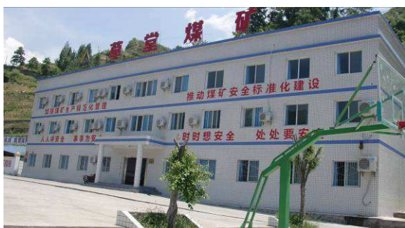
Fig. 6 Administration Building of Caotang Mine
