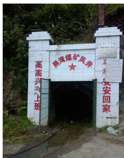
Fig. 11 Ventilation Adit of Heiwan Mine
