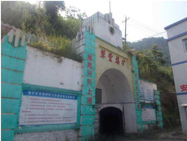
Fig. 1 Primary Transport Adit of Pit No. 1 of Caotang Mine
