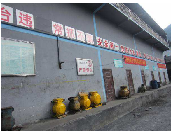
Fig. 25 Repair Workshop and Storage of Changhong Mine
