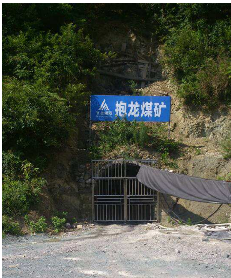
Fig. 18 Main pit portal of Baolong Coal Mine
