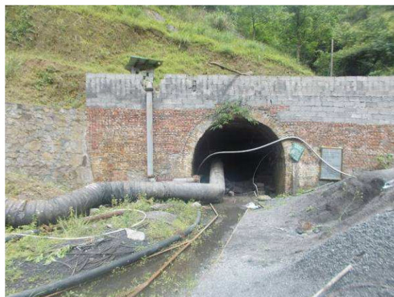
Fig. 22 Ventilation Adit of Changhong Mine
