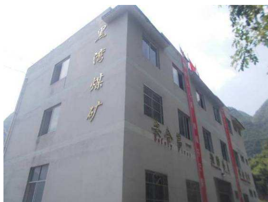
Fig. 13 Administration Building of Heiwan Mine
