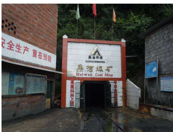
Fig. 10 Primary Transport Adit of Heiwan Mine
