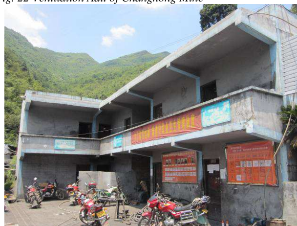
Fig. 24 Miners Bathroom and Store Room of Changhong Mine
