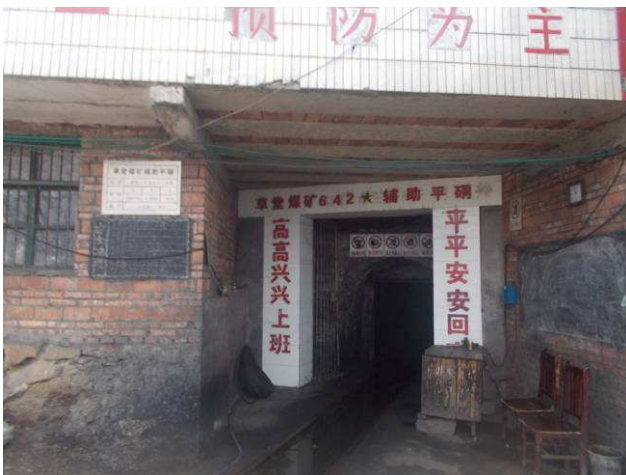
Fig. 3 Primary Transport Adit of Pit No. 3 of Caotang Mine
