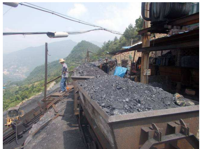
Fig. 4 Primary Transport Adit of Pit No. 3 of Caotang Mine
