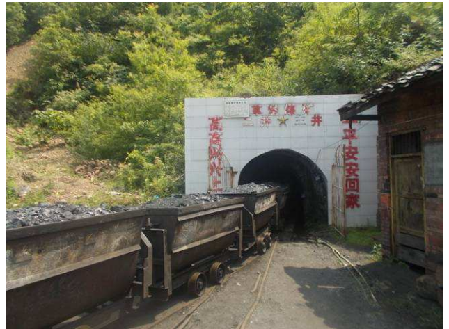
Fig. 2 Primary Transport Adit of Pit No. 2 of Caotang Mine
