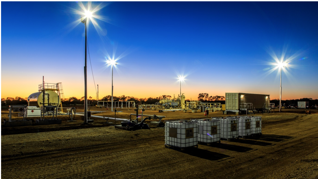
Figure 1: Brewer Estate City Gate Gas Plant
