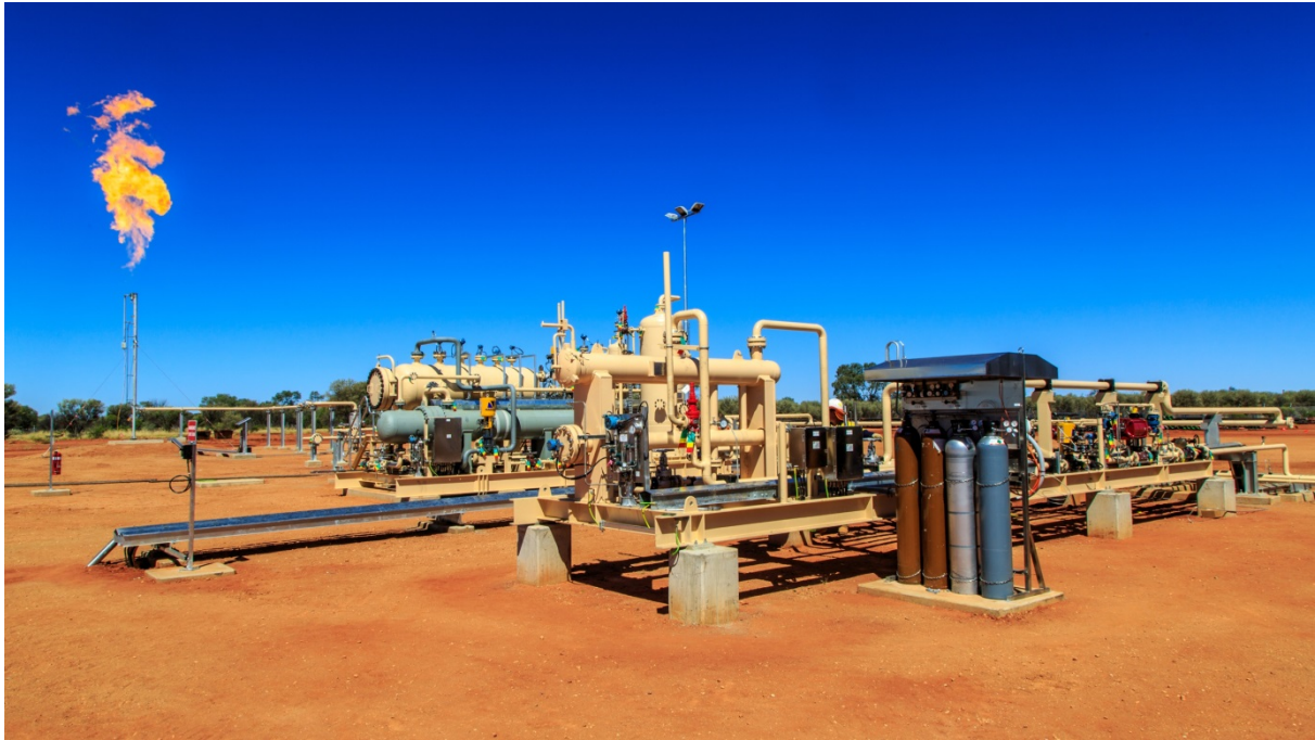
Figure 6: Brewer Estate City Gate Gas Plant being commissioned in March 2015
