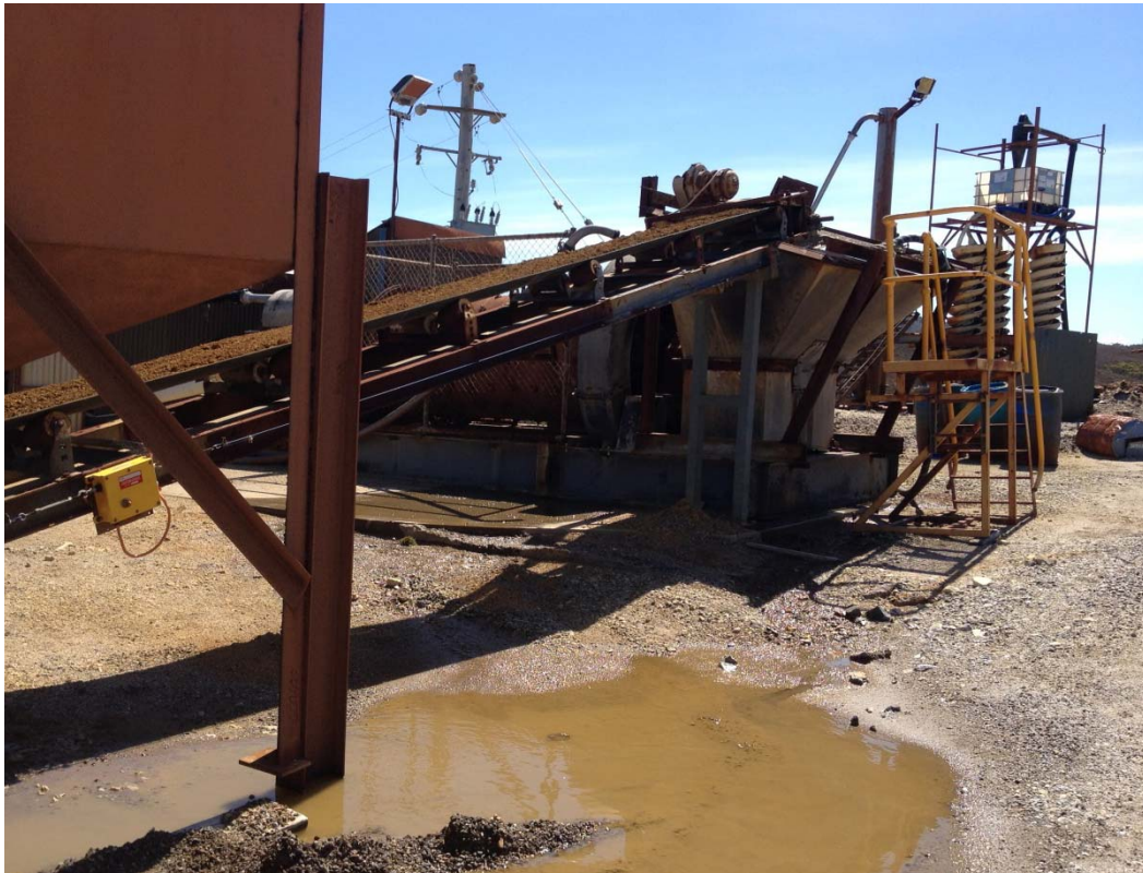
Figure 2: Run of Mine Ore being fed into the ball mill during program of due diligence
