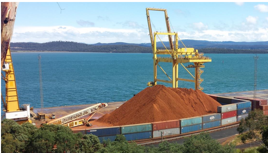
Figure 11: Bauxite stockpile at Bell Bay Port on 26 December 2015. Walls of old containers form a break & stockpile boundary. The rail entering into Bell Bay Port is in the foreground and it connects to the rail immediately adjacent to the bauxite stockpile. Ships will berth at the concrete wharf and be loaded by the large telestacker ship loader at a high rate.
