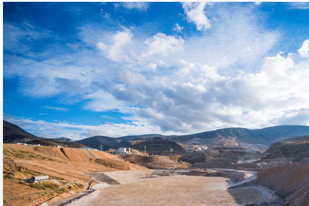
Sulfide Plant Site Earthworks
