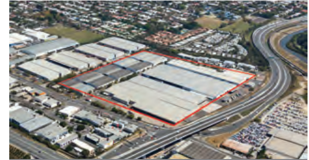
Hendra Distribution Centre
