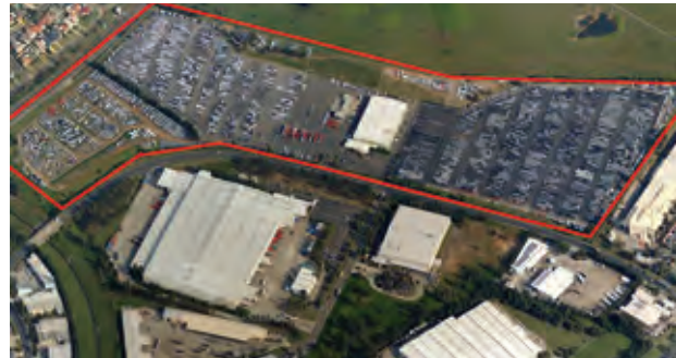
Ingleburn Distribution Centre
