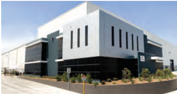
20-50 and 76-82 Fillo Drive and 10 Stubb Street
