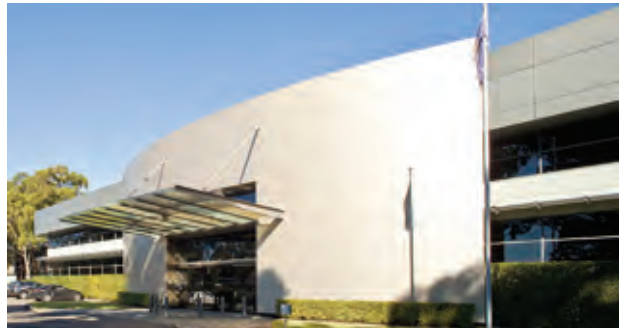
Macquarie Technology Centre
