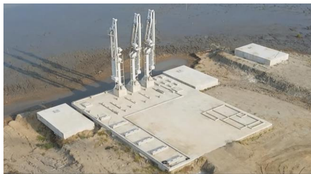
Construction of the Loading Platform
