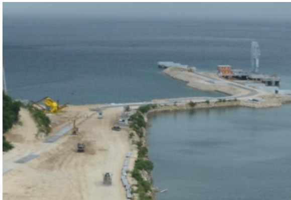
Construction of Jetty
