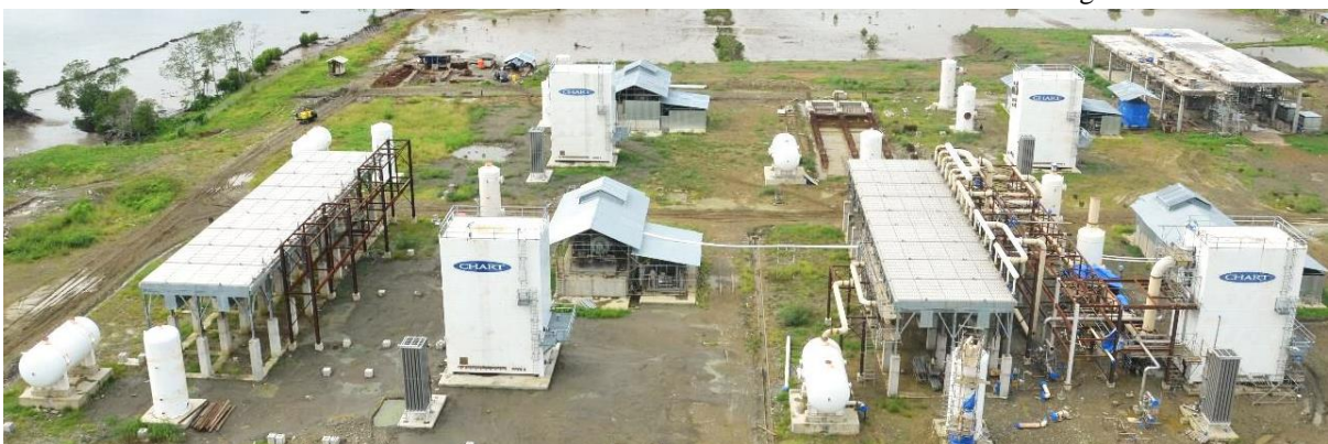
Compression & Liquefaction Trains
