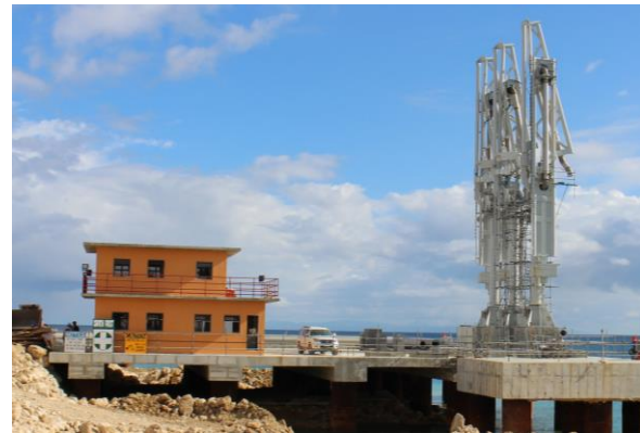
Jetty Deck, Control Room and Loading Arms
