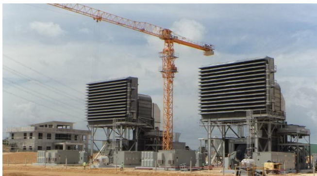
Construction of Power Station
