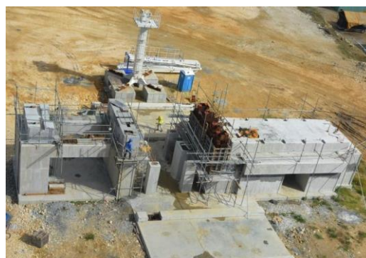
Construction of Power Station
