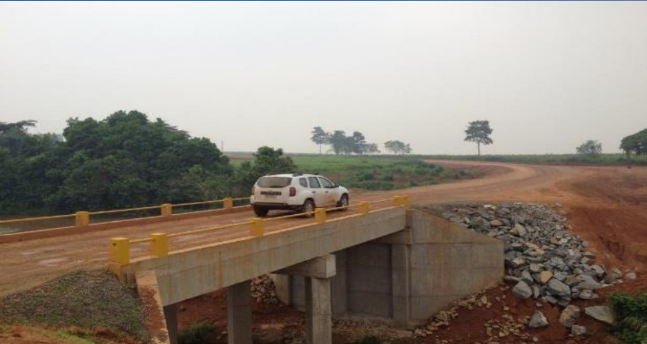
Mine access road including construction of two bridges completed
