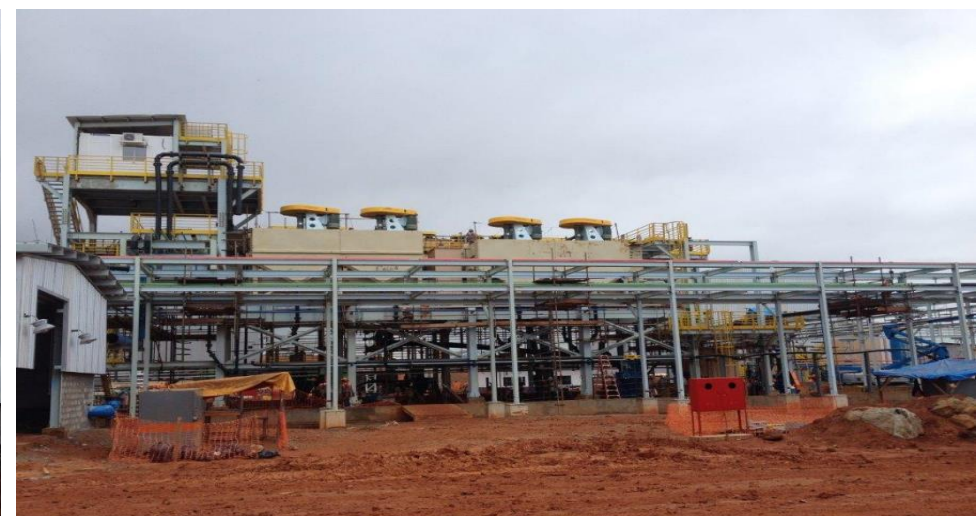
Installed flotation cells and plant control room
