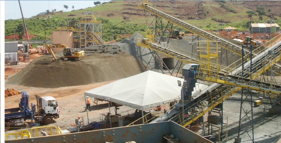
Crushing section now operational
