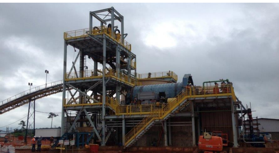
Ball mill, feed conveyor and hydrocyclones installed
