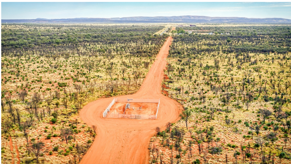
Dingo Pipeline Right of Way; Looking South towards Brewer Estate
