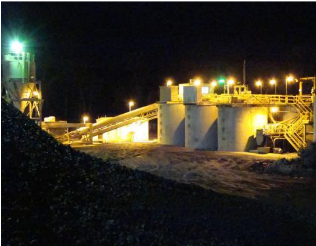
Figure 2. Night view of the Maldon Treatment Plant
