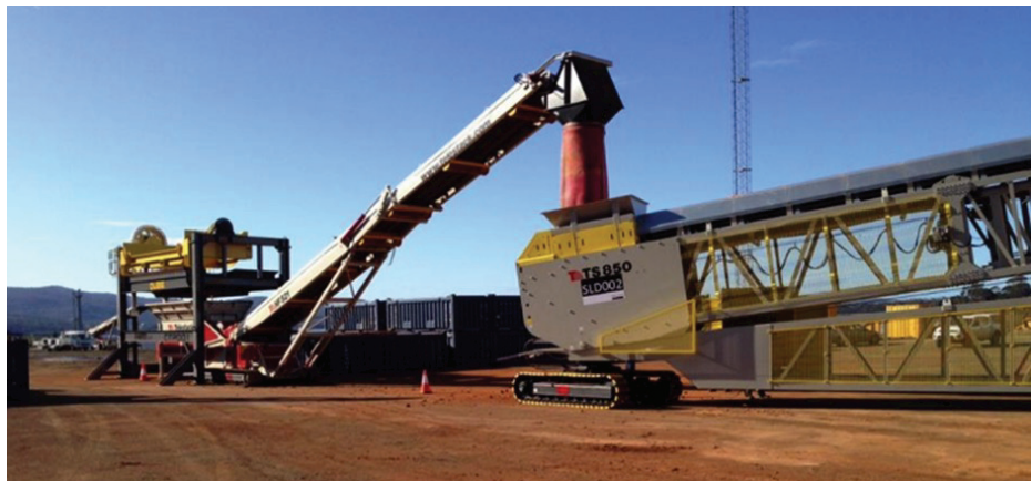
Figure 9: Qube’s tipping frame tips 22 tonnes of bauxite from the rail container directly into the feed hopper of the Telespacer ship loader which also does the radial stacker duties.
