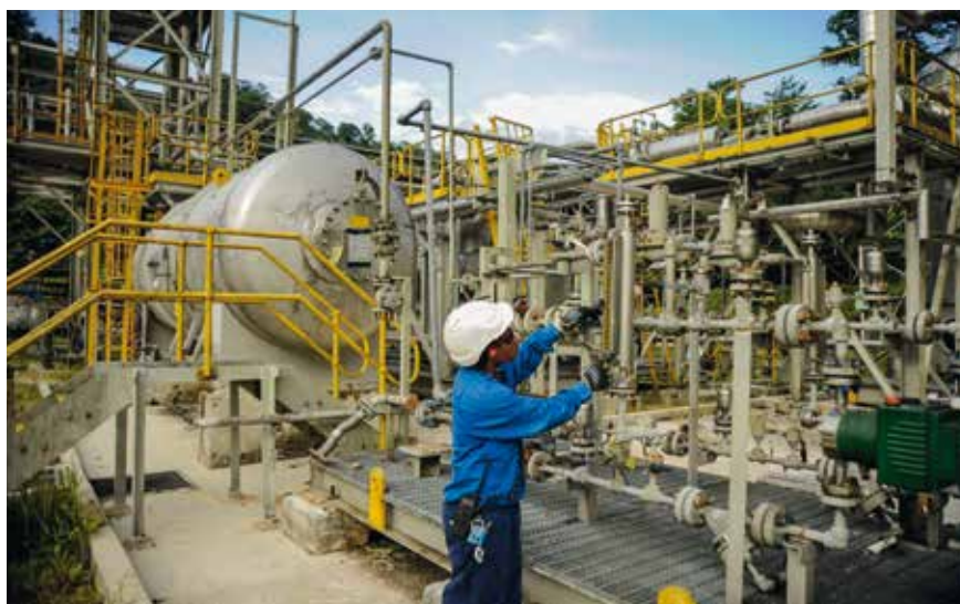
Central Processing Facility, Kutubu, PNG Highlands.
