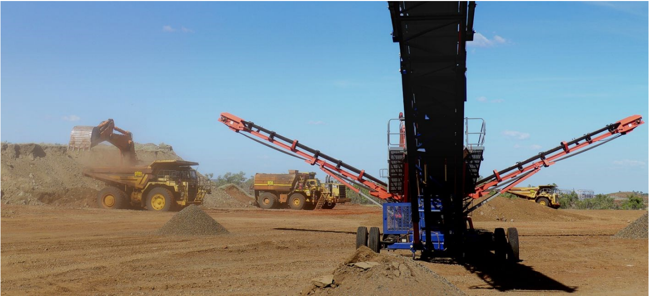
Figure 5: Quarrying and crushing of rock to provide much needed road-base product.
