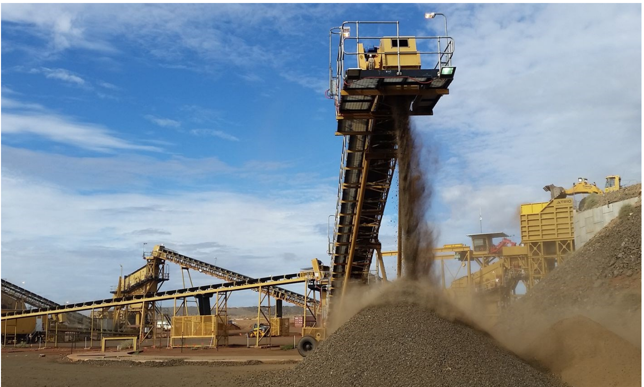
Figure 2: Replacing of the final rolls crusher with a cone crusher resulted from successful test-work using the Company's mobile crushing plant that clearly showed the benefits in separating coarse native copper (+40mm in size), from the associated ore, achieving up to 95% copper concentrate. Top image shows the cone crusher up close and the below image shows commissioning of the cone crusher.
