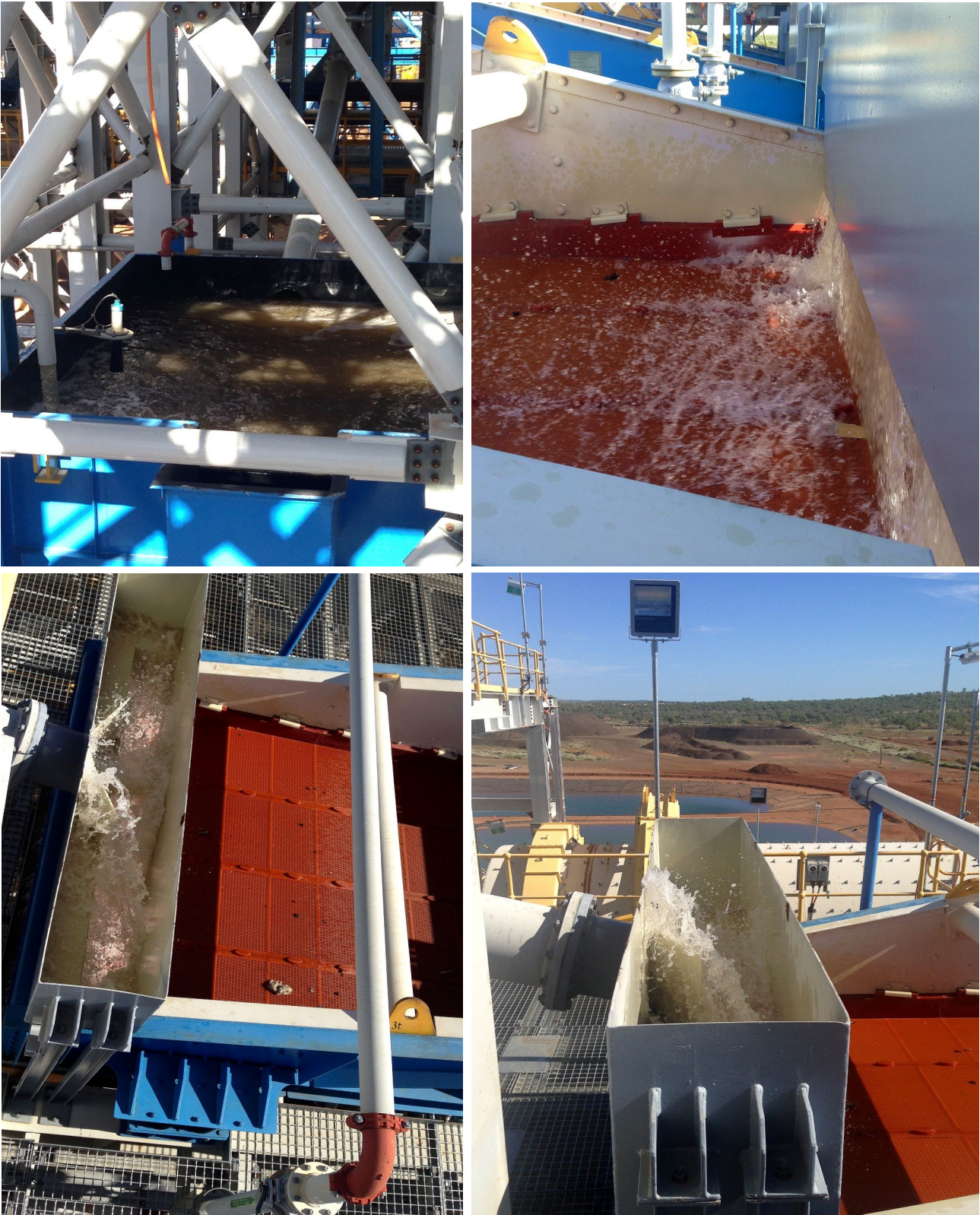
Figure 3: Wet commissioning activities clockwise from top left; Classifying - Fine Screen (2mm) undersize pump box and screen (right); Classifying - Fine Screen (1mm) feed line and feed box; and Classifying - Intermediate Screen (4mm) feed line and feed box.
