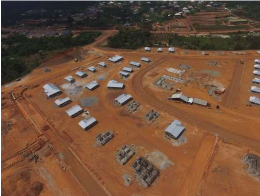
Construction of Relocation Housing – Ayanfuri, Ghana
