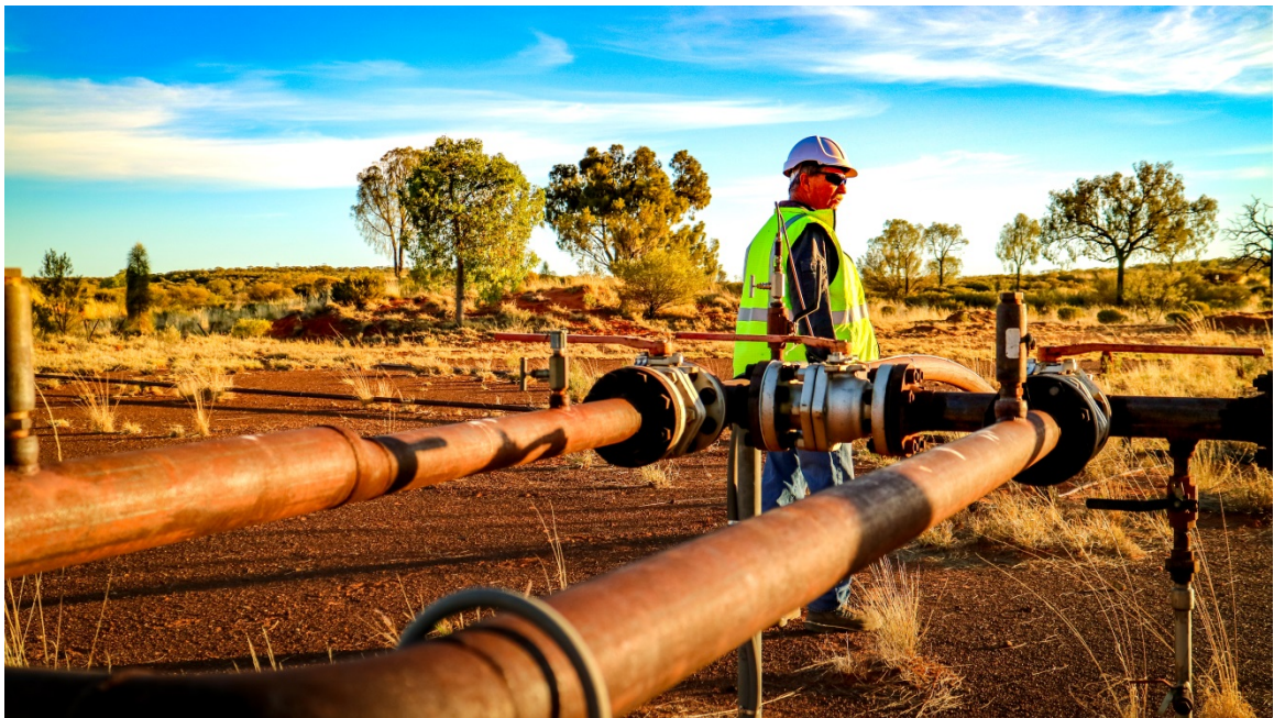
Figure 3: Mereenie; West Mereenie 5 pipe integrity inspection
